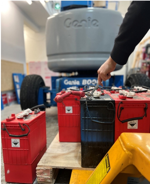
Original lead-acid batteries being removed from genie lift.
