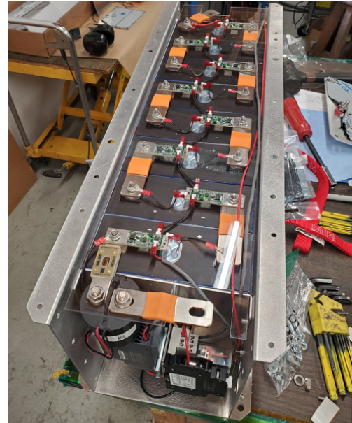
Battery back during assembly process using lithium-iron phosphate modules with a total of 7.2 kWh capacity.
